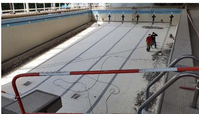
Figure 6. Piquage carrelage bassin
