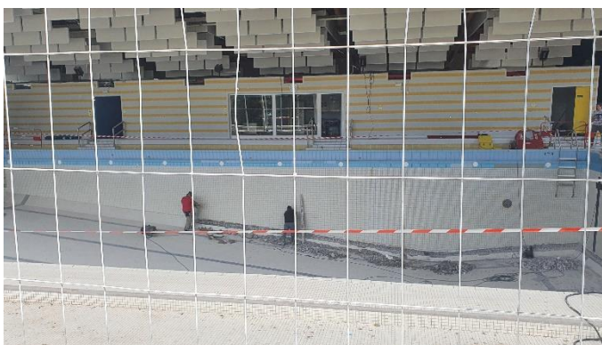
Figure 4. Piquage carrelage bassin
